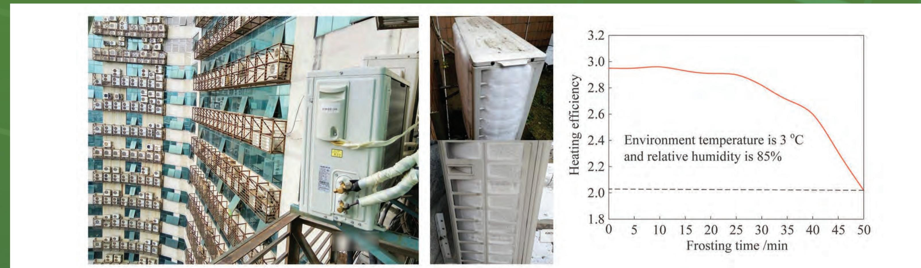
Fig.1 Frosting on the outdoor heat exchanger of ASHP impacting the heating efficiency
