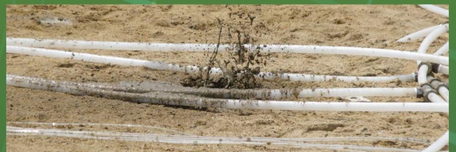
*Vacuum Preloading with Pneumatic Fracturing in Operation (Depth of air injection: 18m)*
