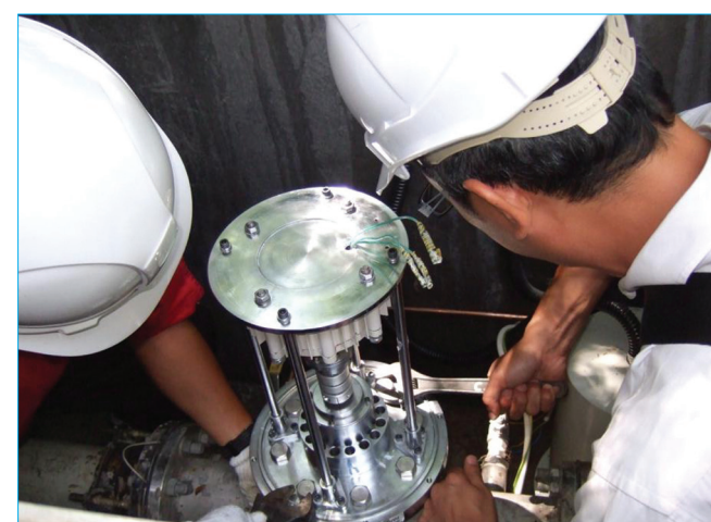
採用微型發電機，適合在狹窄的地下水管空間安裝 The hydro generator system is compact for installation in the narrow underground space of water mains pit
